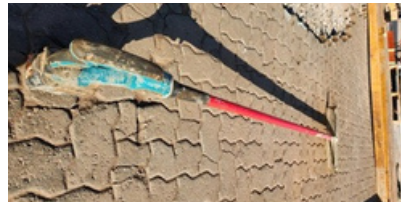
Concrete Rake with Makita Battery Vibrator
